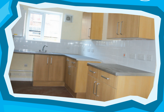
Above: Renovated kitchen, Tyldesley Street.
